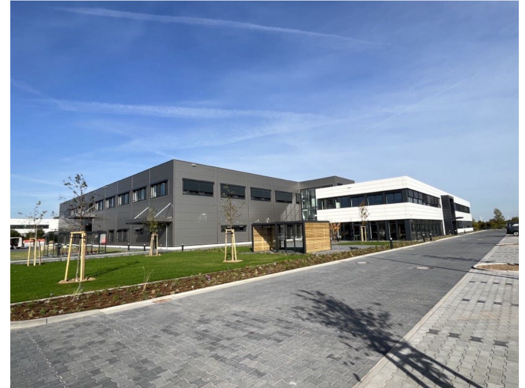
MMG's New Head Office Factory (Germany)
